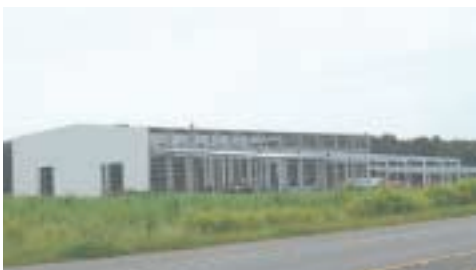
Construction progresses at rapid pace. Picture taken August 1, 2006.
