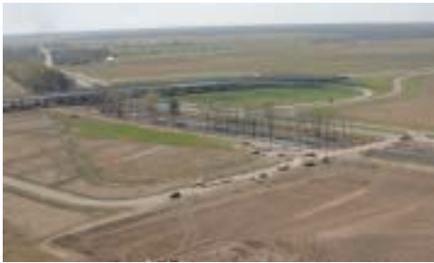
Facility located at intersection of Hwy. 90 and La. 311. Picture taken March 1, 2006.
